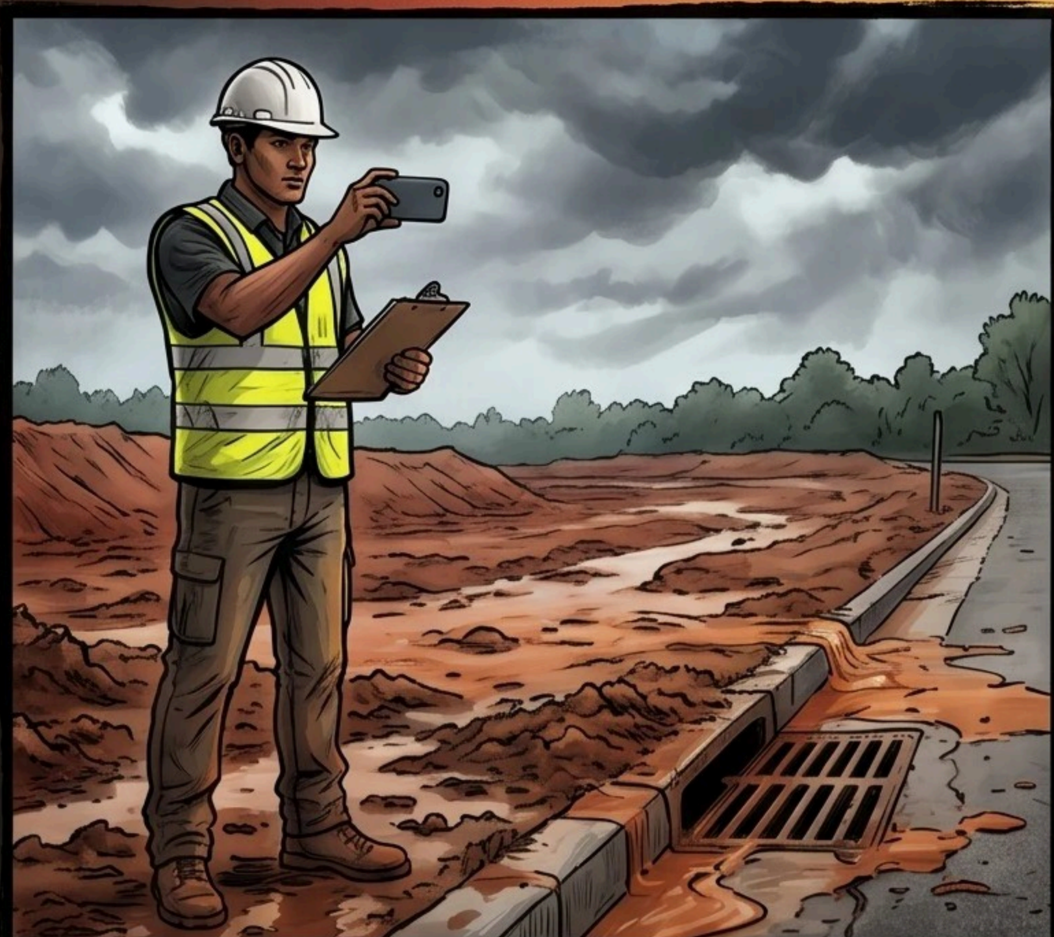
WEDNESDAY -- DEMLR INSPECTOR. NOTICE OF VIOLATION.
